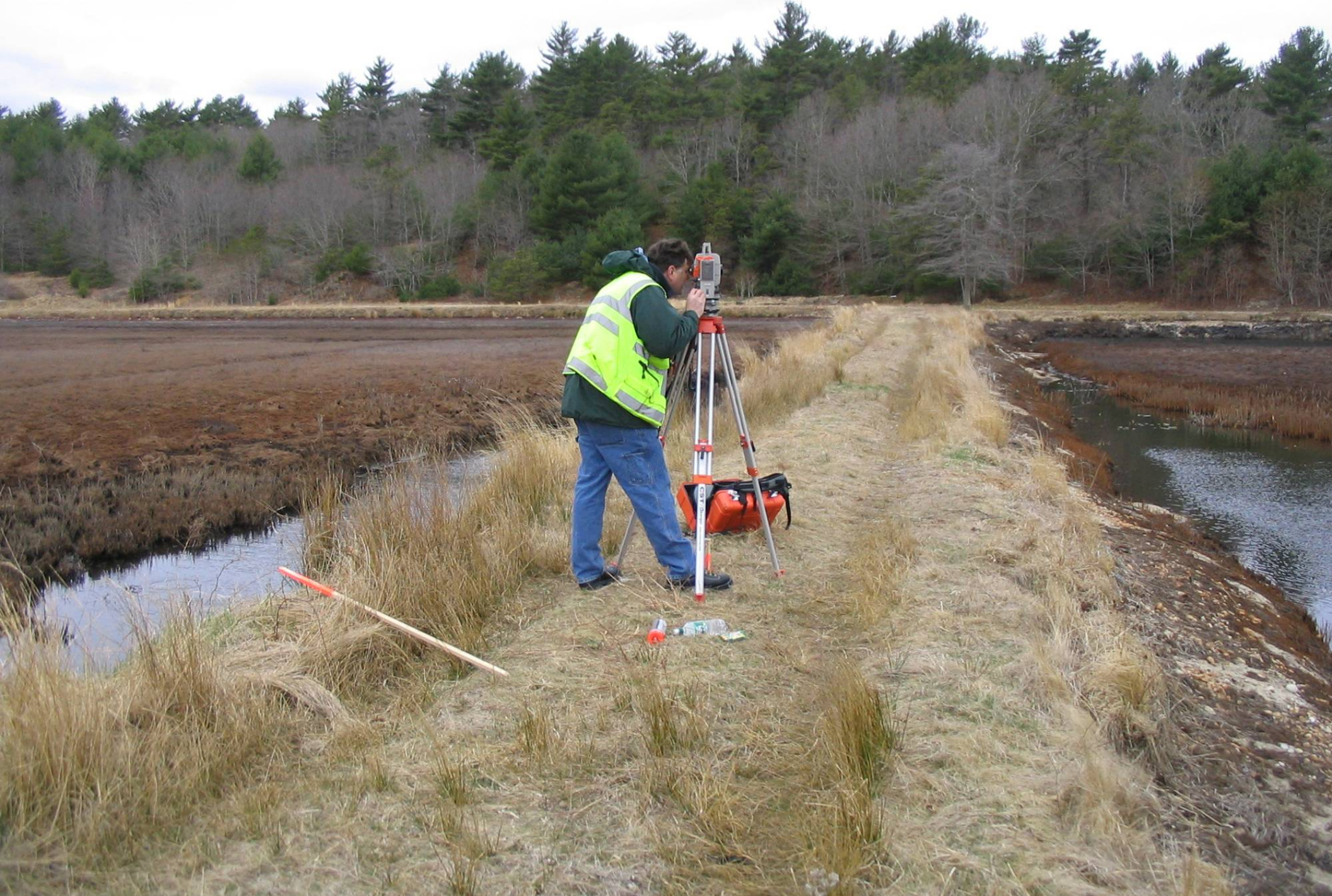
Looking west along Bog 6/7 berm
